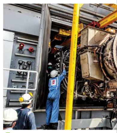
The ten day shutdown started on 10 March 2021. The first step was to carry out physical isolations for plant's declassification. It was done successfully within 4.65 hours, which itself is a benchmark. Around 300 jobs were planned in this shutdown and all these jobs were safely handover, supervised and executed successfully. Apart from Gas Turbine (GT) Replacement, GT Alternator Major overhauling (MOH), NGBC-A overhauling and HRSG inspection were major jobs.
